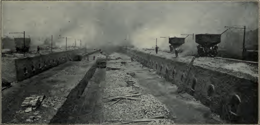
FIG. 167. — Coke ovens near Pittsburg. Each of the small doors leads to an oven where the coal is burned and changed to coke.
